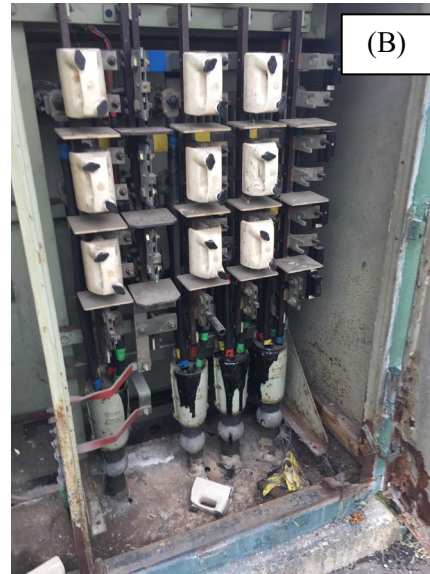
CABLE TERMINATION, (A) "BANANA BOX", (B) "BAGPIPE". BOTH VARIANTS HAVE BEEN ASSOCIATED WITH DISRUPTIVE FAILURE ARISING FROM COMPOUND TERMINATIONS
