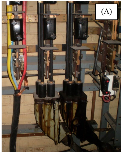
CABLE TERMINATION, (A) "BANANA BOX", (B) "BAGPIPE". BOTH VARIANTS HAVE BEEN ASSOCIATED WITH DISRUPTIVE FAILURE ARISING FROM COMPOUND TERMINATIONS
